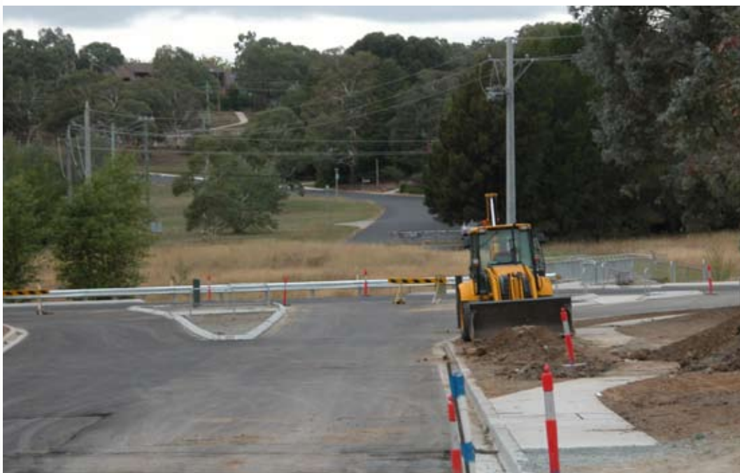
New road infrastructure—kerbing, barriers, footpath, drainage and pavement
