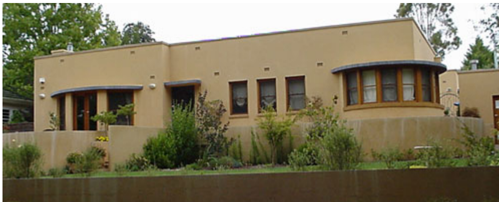
Figure 1. Front view of 24 Arthur Circle, Forrest.
